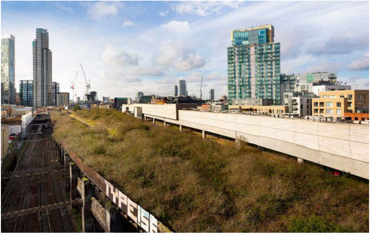
Aerial view looking south over platform level
