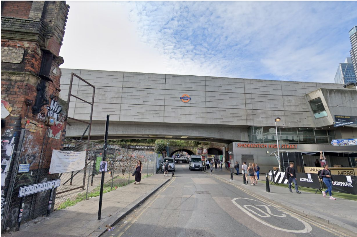
View south down Braithwaite Street
